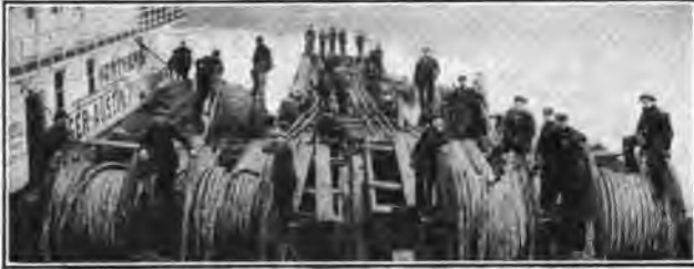
Duquesne Light Co. laying 11,000-volt Submarine Cables made by Standard Underground Cable Co. across Ohio River at Pittsburgh.
